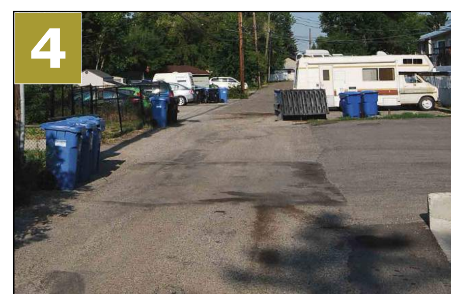
4 Lane condition along northern site boundary
